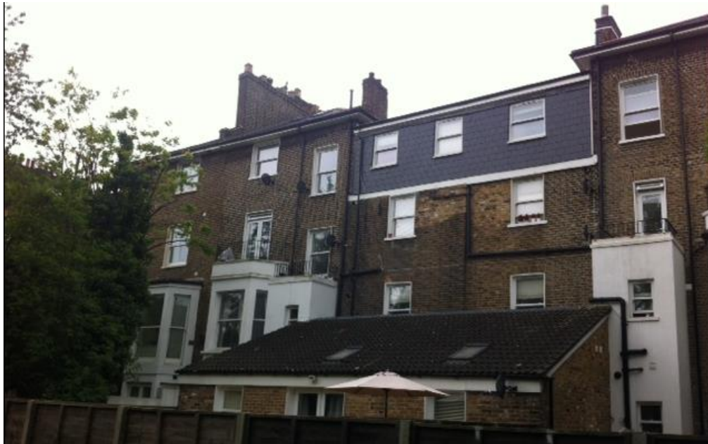
Image 6: Existing rear elevation of No.13-17 Thane Villas
