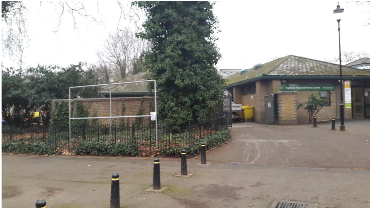
Image 2: View of front (south) elevation
